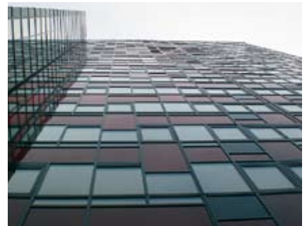
5) Extra prize for small-scale renovation (Non-Residential) Elsa Morante Public Library, Lonate Seppino, Italy DAP Studio architects, Milan Contractor Gruppo EDILIA, Turin.
