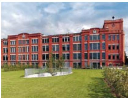
4) Jury prize for Energy Efficiency (Residential) De Torenflat, Zeist, The Netherlands Frowijn de Roos Architecten, Zeist Kremers Aluminium, Tilburg.
